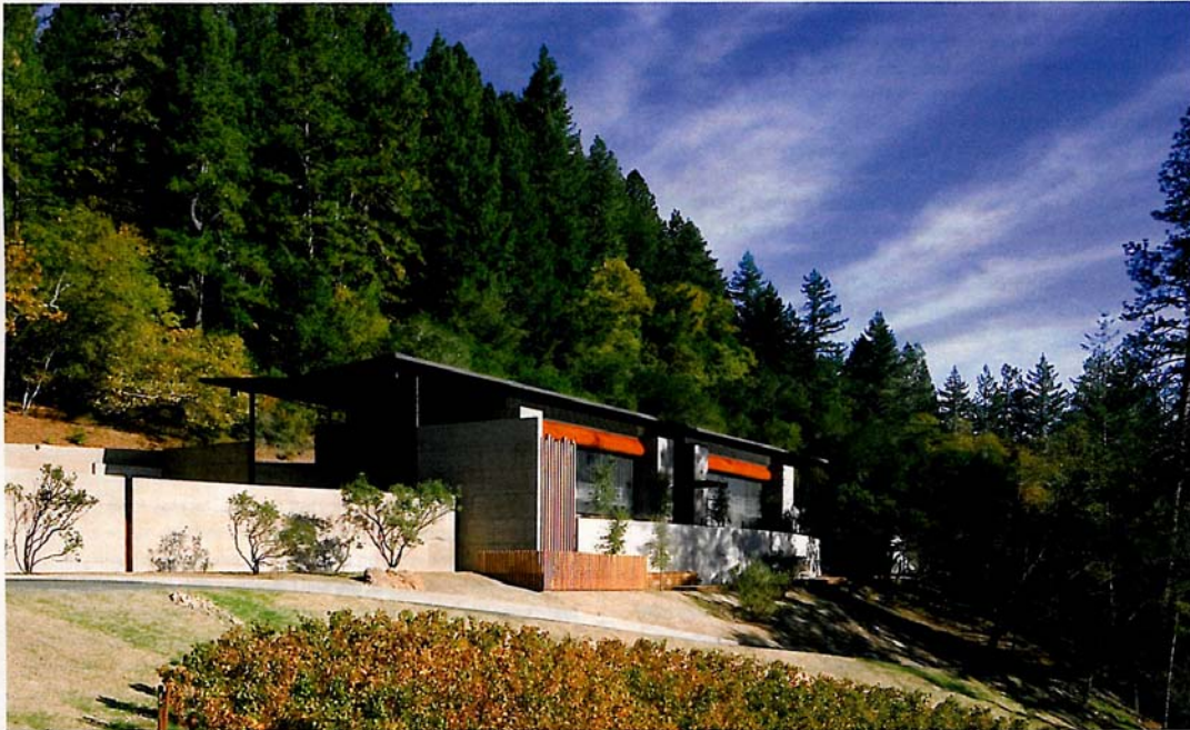
Rising above Napa Valley proper is Howell Mountain, home to Cade, a winery where going green is paramount—including the use of a special concrete made from recycled materials.
